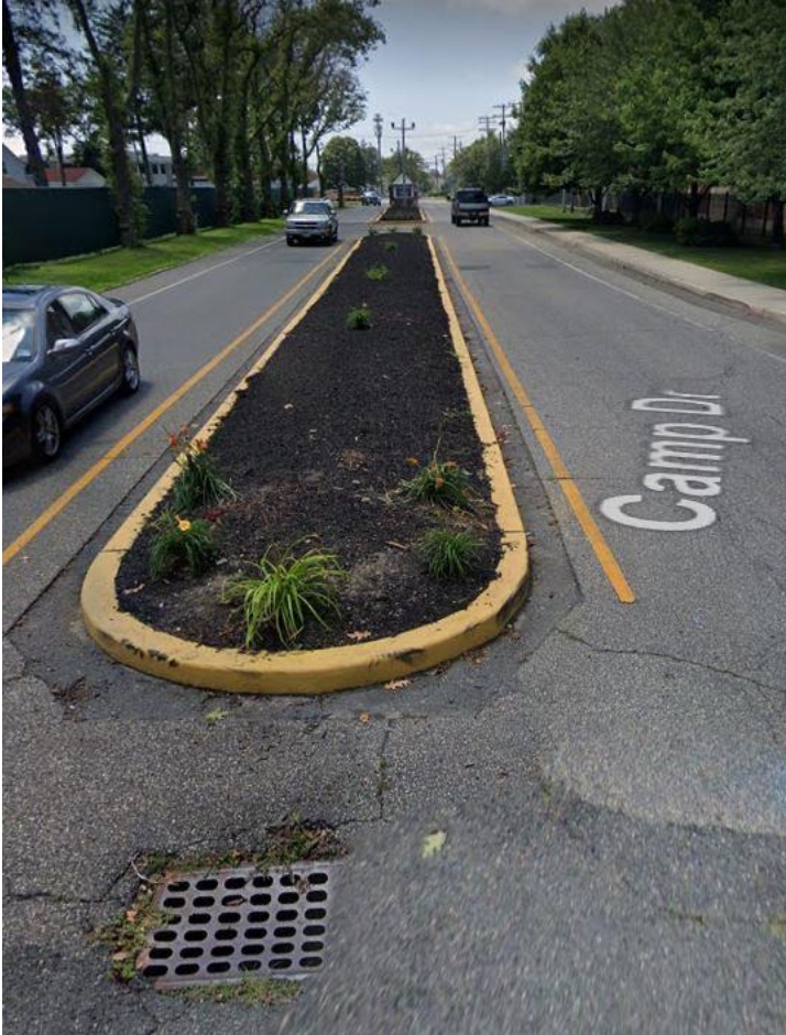
Photo 1: South Facing view of the median along Camp drive.
