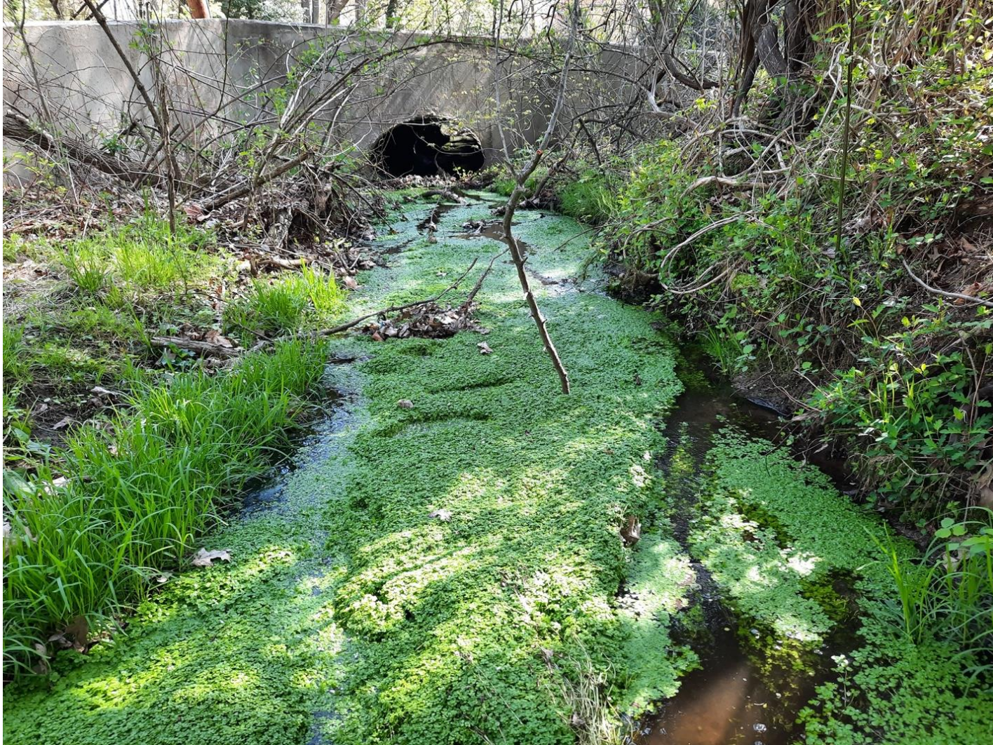
Photograph LVLS1: A photograph of a portion of the GLIN survey area of the Little Shabakunk Creek Tributary at the Lawrenceville NJDMAVA HQ taken on April 19, 2021. This photograph shows the site conditions of the beginning portion (lower bounds) of the surveyed stream segment.
